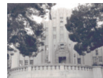
1900 Cochise County Courthouse
