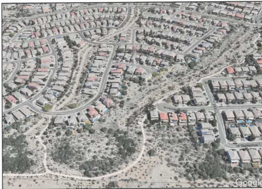
Before Condition - Common Area within Parcels C & D (South of Shaughnessey Rd) Note – Walking Paths Connect Two (2) washes
