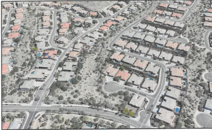
Before Condition - Common Area within Parcels A-1 & A-2 (North of Shaughnessey Rd) Note – No Walking Paths
