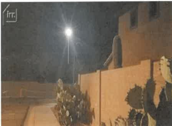
View of Freeway Lighting near 27th Avenue & Cedarwood Lane
