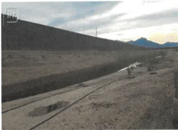
Sound Wall & Buffer Area
